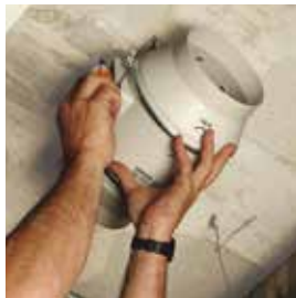
Place the impeller and motor assembly.
