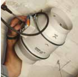
Carry out the wiring connections.
